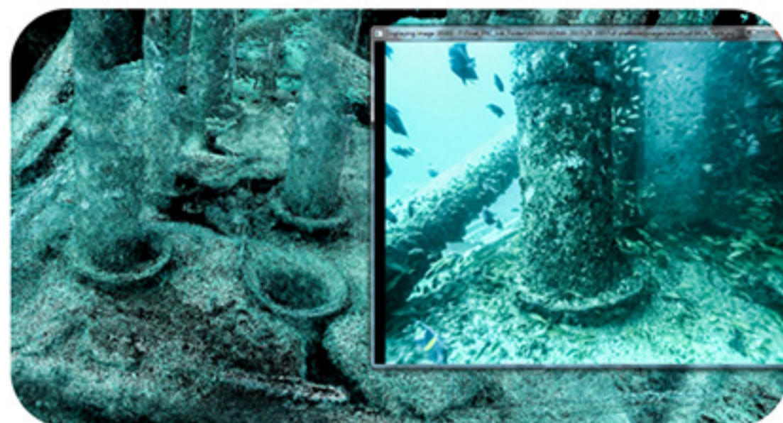
Conductor lack of Centralization
